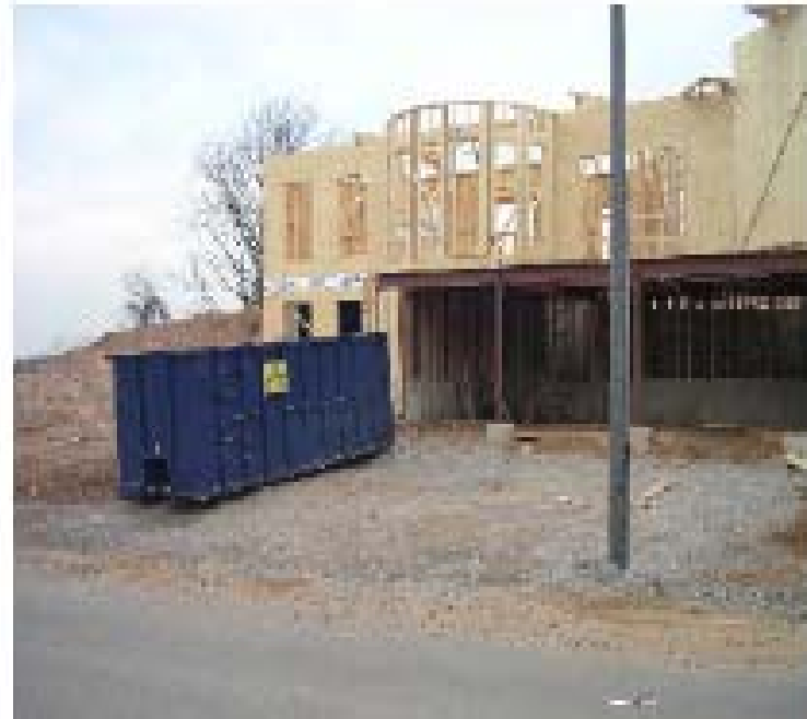
New residential construction
