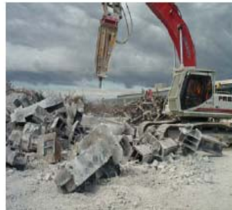
Concrete recycling: major demolition
