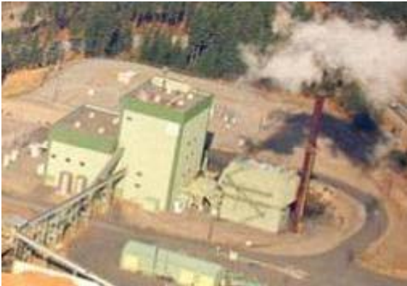
30 MW ABB/Zurn biomass plant, CA
